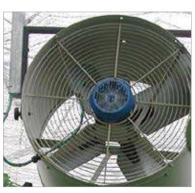
Horizontal Air Flow (HAF) fans are used to circulate air within the greenhouse.
