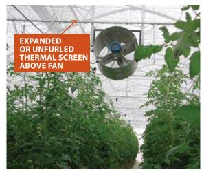
Thermal screens offer a flexible and efficient way of managing the greenhouse environment.
