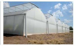
The natural 'chimney effect' of rising hot air and falling cooler air which is the basis for passive ventilation becomes truly effective above approximately 3.5 metres. Beyond this, the movement of air over the greenhouse provides the main venting action which is why roof vents are superior.
