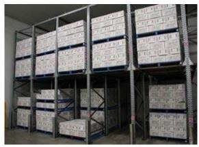
Rack systems allow efficient use of cold room space as well as good air circulation around stacked produce.
