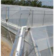
Venting (preferably insect proof meshed), of sawtooth designs can be limited by wind direction and must be sited correctly.
