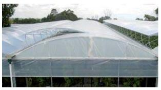
Unmeshed single roof vents on open-ended multispan.
